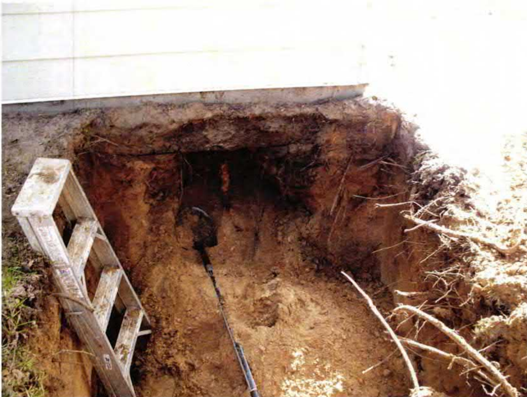
Picture 2: UST 408Elderberry removal in progress. Vent line under building.
